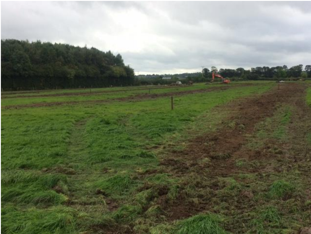
Picture 3. Drainage on the Derrypatrick farm
