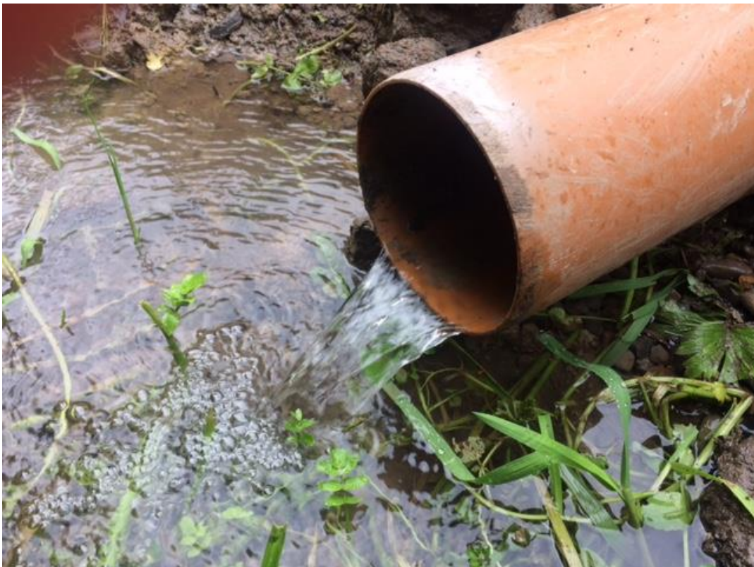
Picture 4. Flow of water from the outlet pipe following drainage
