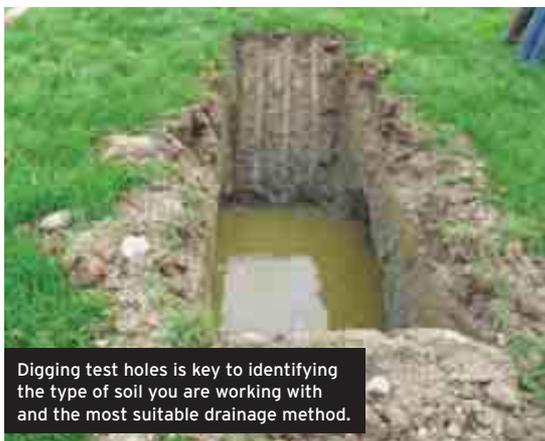
Digging test holes is key to identifying the type of soil you are working with and the most suitable drainage method.
