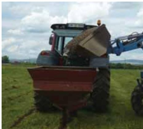
Figure 1. Gravel filled mole drainage
