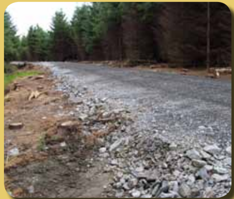
Completed harvest road
