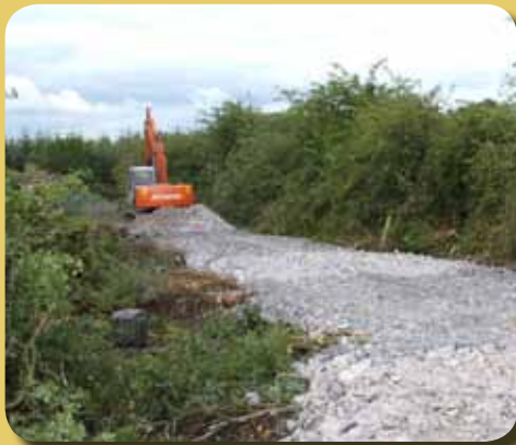
Build road in dry weather
