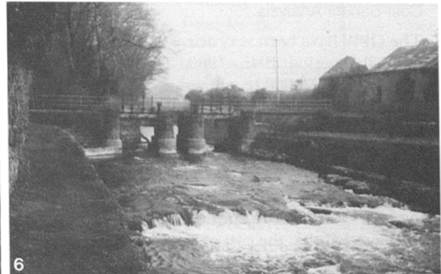
Figure 3. Design for flashfloods. A larger cross-section allows a greater increase in flow for a given increase in head.
