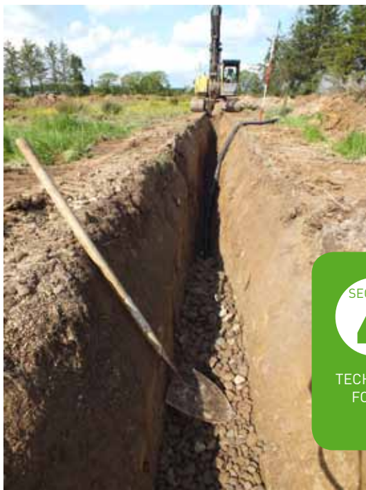
Figure 2. Drainage trench excavation
