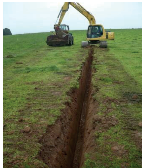
Fig 1b. Drainage trench excavation
