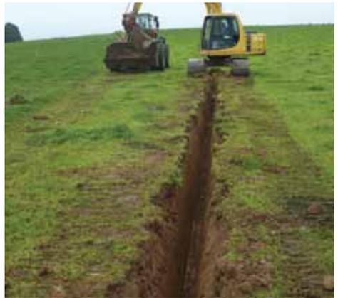
**Fig 1b.** Drainage trench excavation
