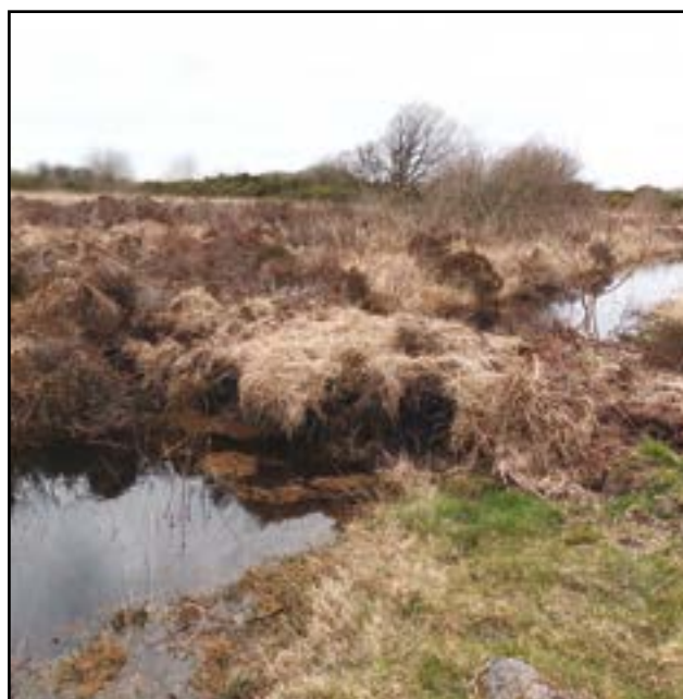
Drain one week after installation of dams
