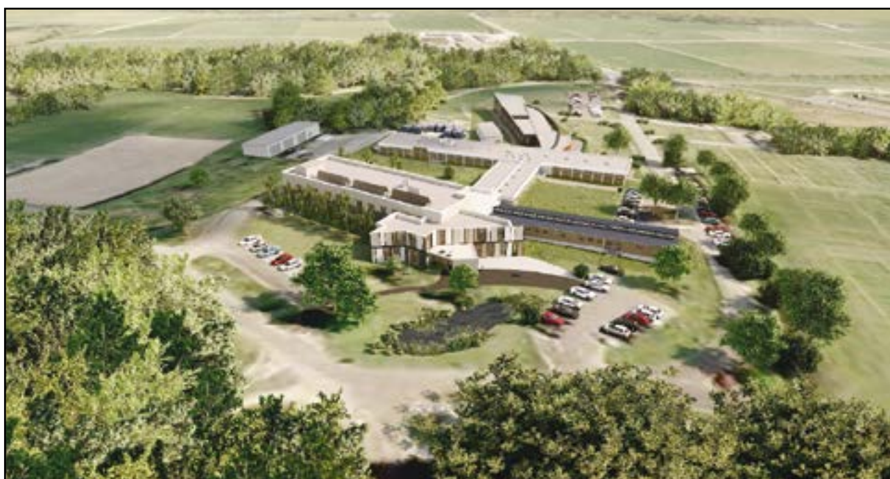
Figure 2: The New National Agricultural Sustainability Research and Innovation Centre currently under construction.
