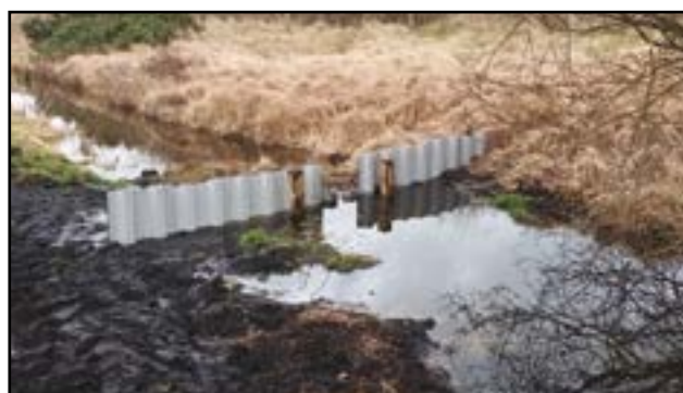
Drain one week after installation of dams
