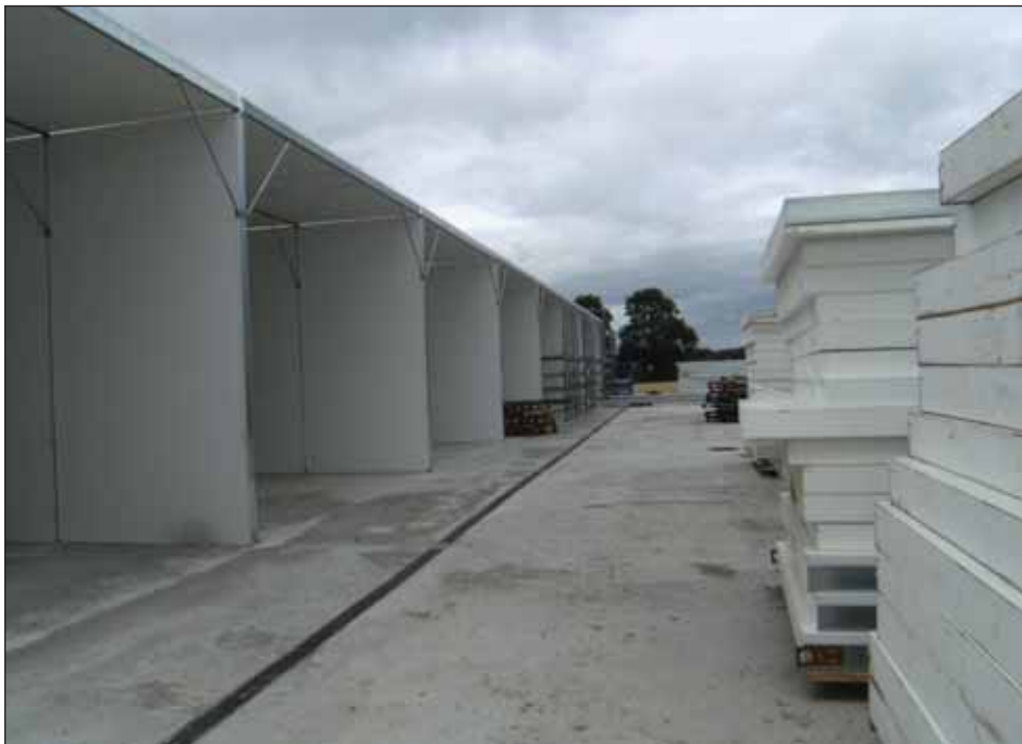
A new high insulated mushroom growing unit made from reinforced panels. The modern unit is located in Tullow, Carlow.
