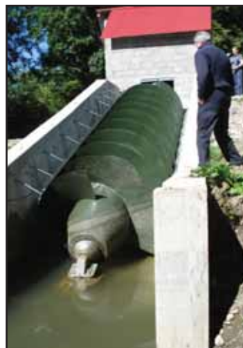
The Archimedes Screw now used for over 2,000 years as a pump is becoming a popular technology choice for low-head hydro-power generators. Source F O'Brolchain
