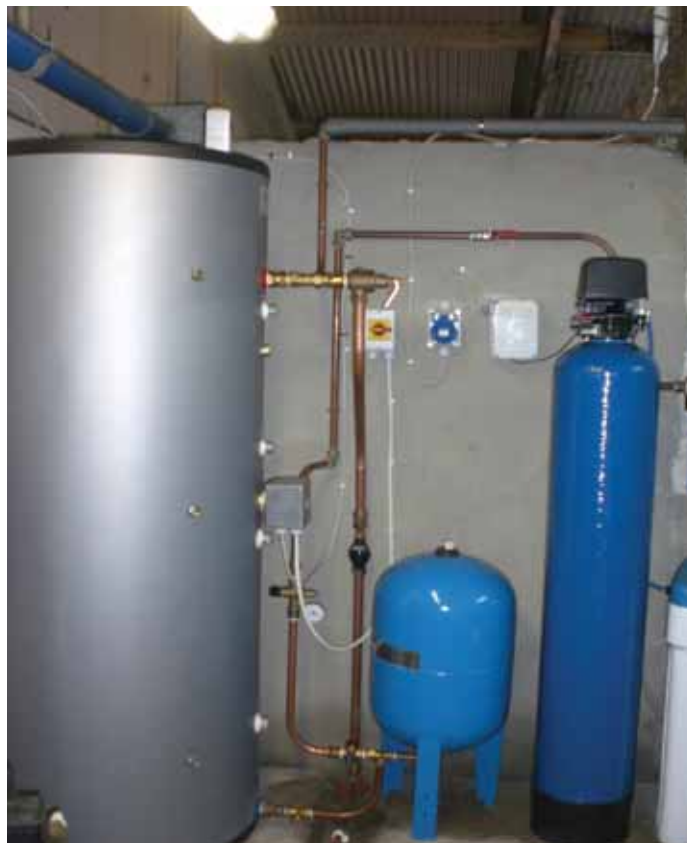
3 kW Electrical heating immersion system with water softener. Note pipes should be lagged.
