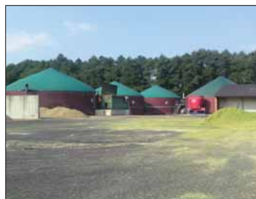
Farm scale biogas plant in Germany, co-digesting maize silage and pig slurry.
