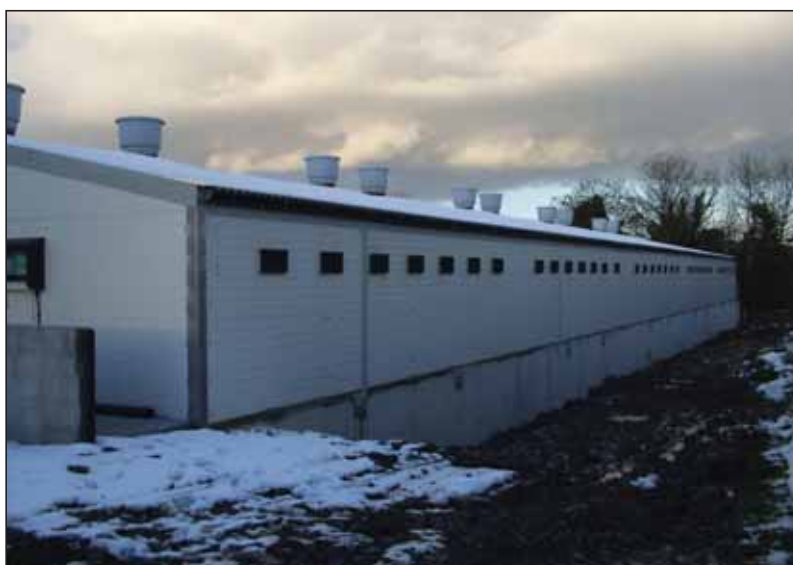
A well insulated building - notice snow not melting on roof.
