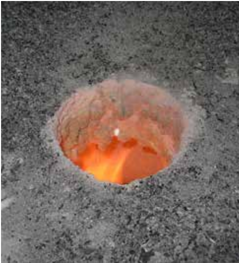
Clinker formed on the grate of a boiler
