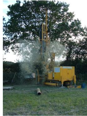
**Figure 1** Installing groundwater monitoring points.
