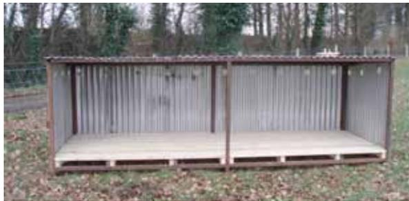
**Figure 1.** Steel roofed shelter, providing both wind and rain protection
