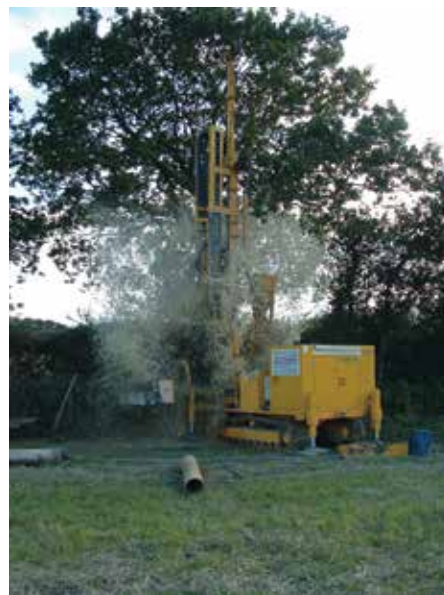
Figure 1 Installing groundwater monitoring points.
