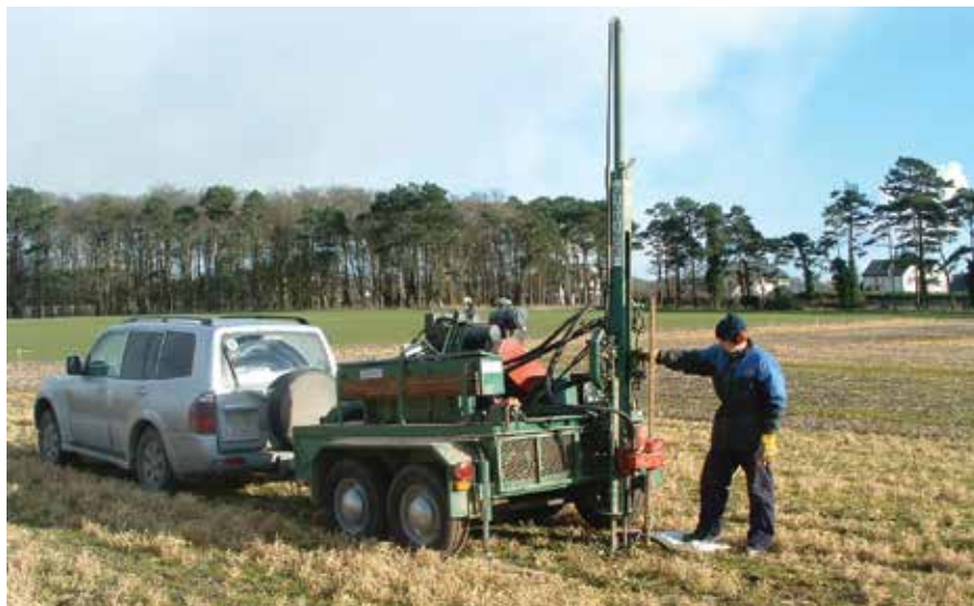
Installing groundwater investigation wells.
