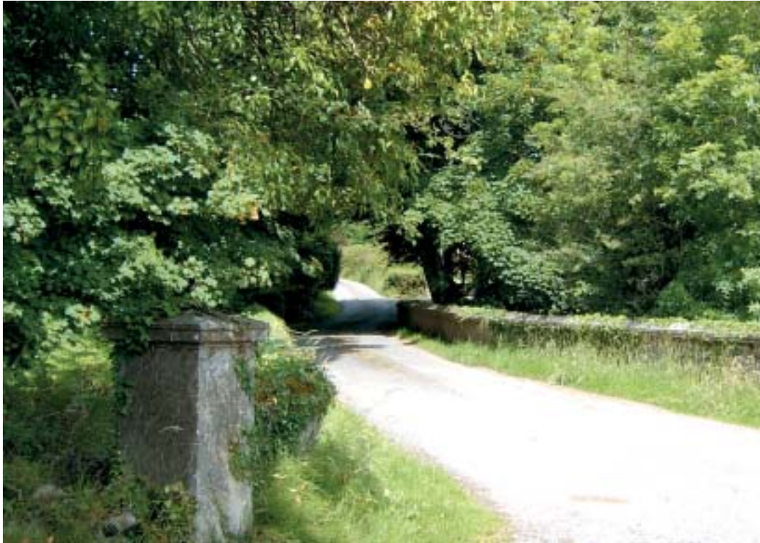
A minor road in Co. Tipperary. (Photo: John Devane)
