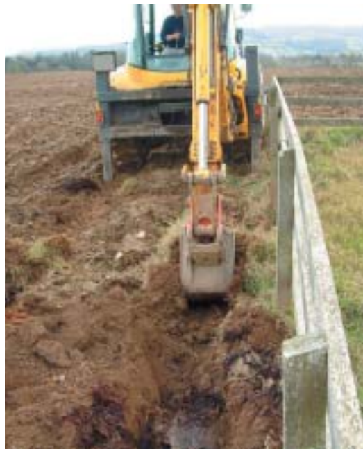
Digging the trench (Photo: Catherine Keena)
