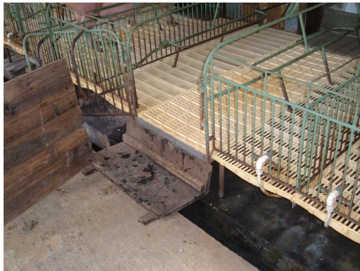
Figure 2. Raised slatted floor and step covering the channel that takes urine and moisture away
