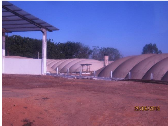
Figure 11. Biogas collection behind weaner and finisher section
