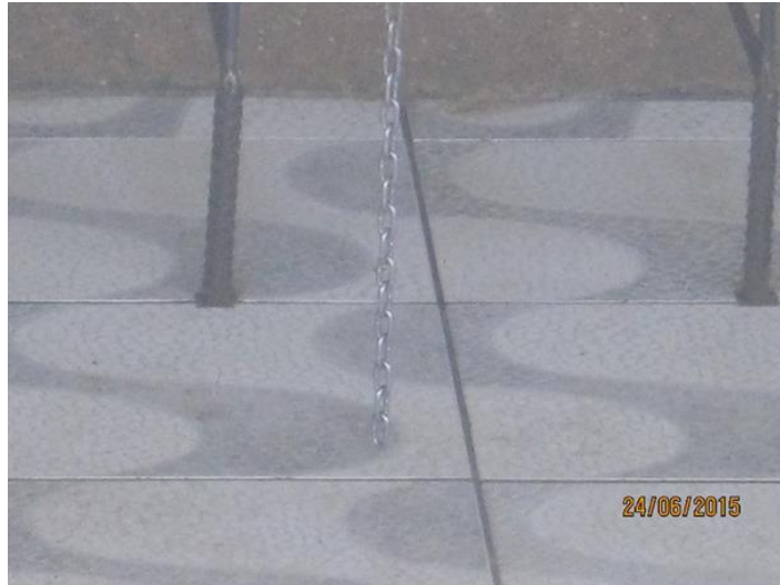
Figure 5. Close up of non-slip tiles in loose dry sow pens
