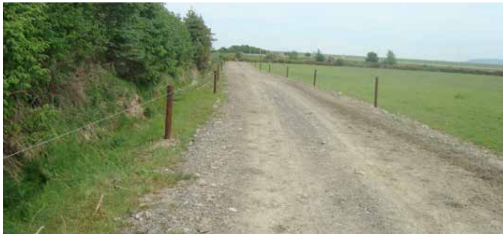
Picture 3. Farm roadway with some loose surface stones - not suitable for cow traffic
