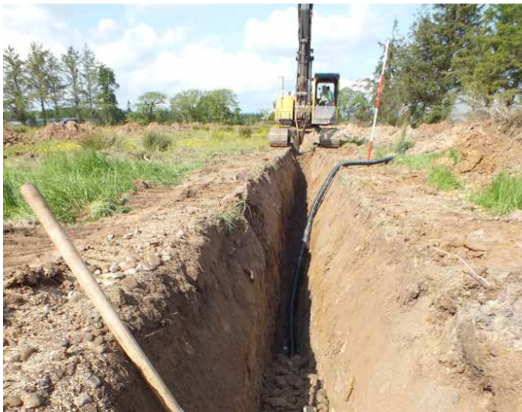
Picture 24. Drainage trench excavation
