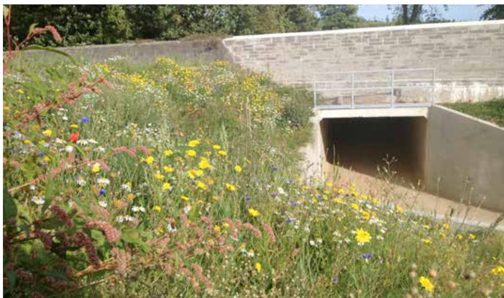
Picture 30. Planting banks with grass and wildflower mixes helps stabilise the banks, prevents undesirable plant species from encroaching into the field, and also provides a habitat for plants and animals
