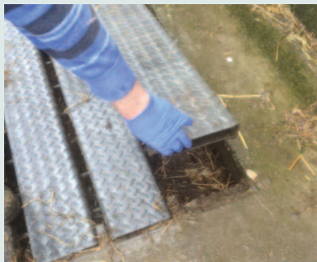
Close slurry openings.
