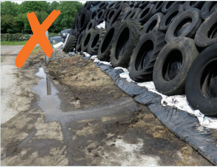
Effluent channel is either absent, blocked, or ensiled grass was filled out over the effluent channel.
