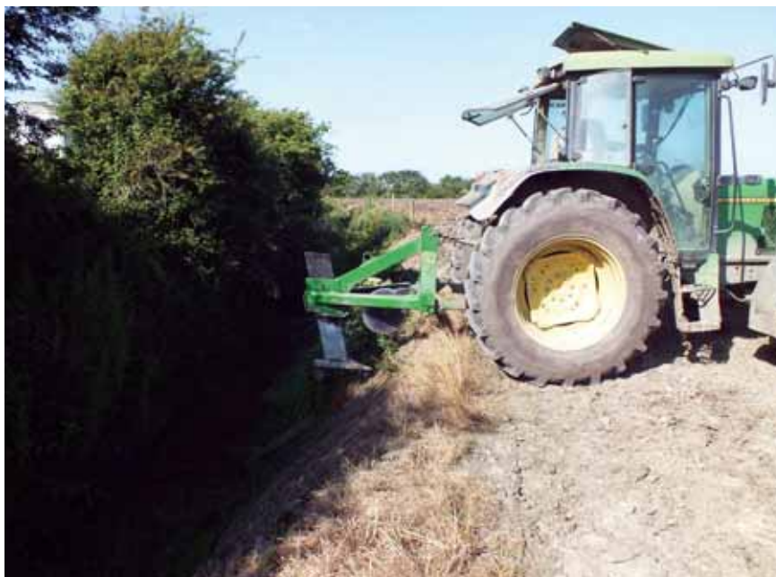
Installing mole drains.
