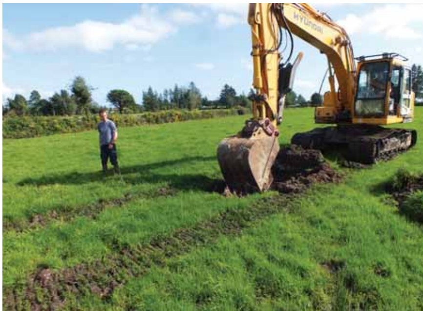
Excavating a test pit.
