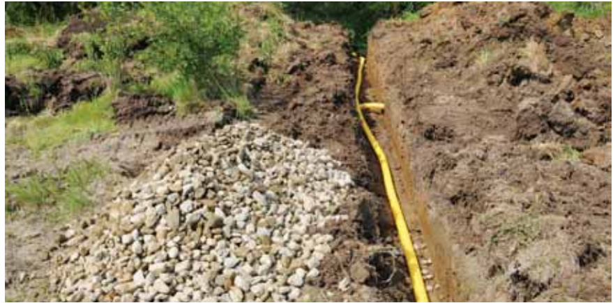
Installing field drains.
