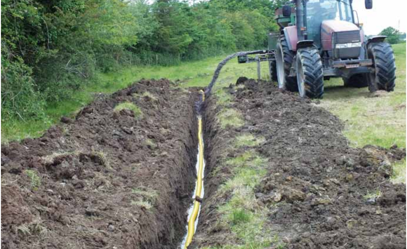
Adding stone aggregate to a field drain.
