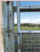
period' can arise causing animals to stray. Use of a gate-stopping device (see picture) to stop a gate swinging outwards is also a worthwhile safety device along public roads.
