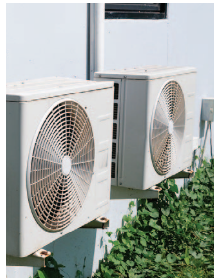
Air-source heat pumps can heat water to temperatures of 55°C.
